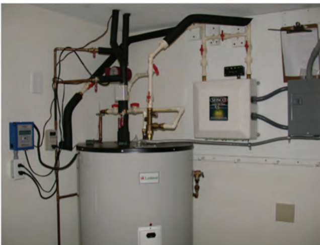
This solar water-heating system, installed on a Florida house, serves six to seven people on average. The storage tank, the controls and the electric tankless heater are shown in the lower photo. Note the subpanel to the right of the heater.
